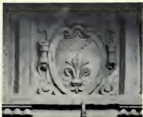
17. - Palazzo Borghese. Portal, center metope (detail of Fig. 16).
